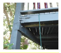
Parts of the handrail to this area is also loose and rectification/repairs are required for safety reasons.
